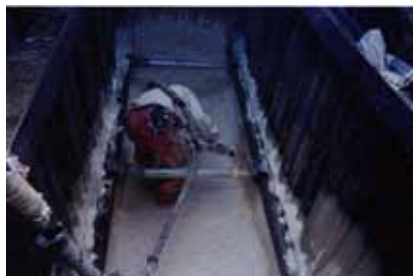
spraying polyurethane by a jet gun
