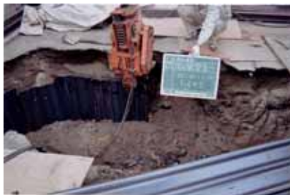
steel sheet pile are driven
