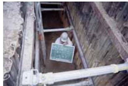
excavation of 4 m
