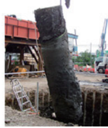
Fig. 15 Test trenching situation.
